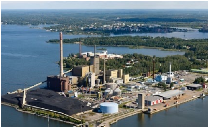
Finland – 140MW CHP – Combined power and heat Forest residue
