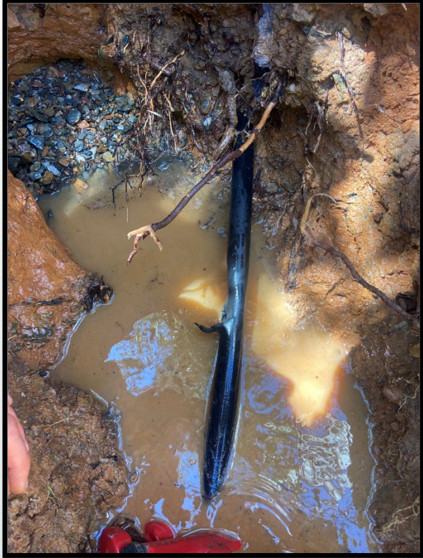
Leak caused by a contractor who was boring next to our line. It was marked out by us for their USA.
