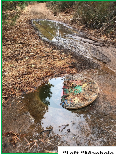
“Left “Manhole Lid was off when Staff arrived, “right”-debris found in manhole causing the backup
