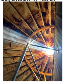
evaluation of corroded areas was necessary prior to sandblasting. It has been initially determined that no such additional evaluation is necessary, based on the small amounts of corrosion related structural issues. Good news!
