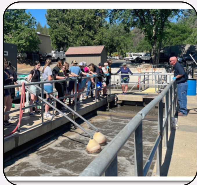
Chief Plant Operator giving a tour of the District's sewer treatment plant to local middle school students
