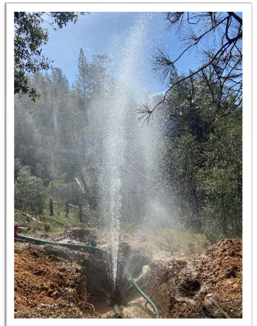
Dewatering the mainline for valve replacement.
