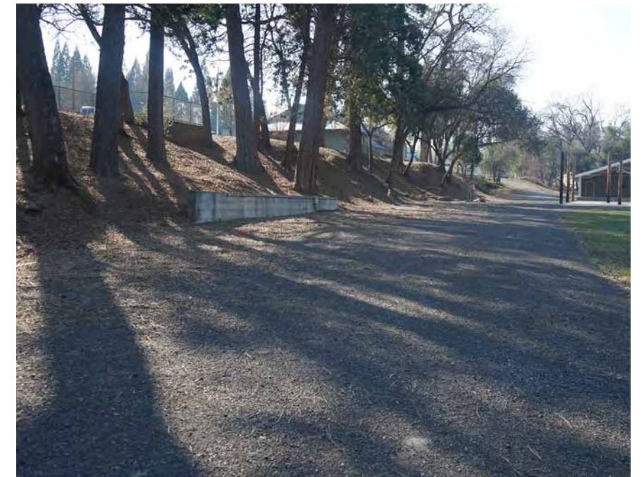
Remove old foundations / abrupt grade changes.
