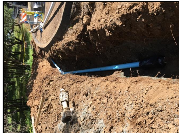
On left you can see the spilt going into the coupling on the right is the completed section with 4" C900 with 45 degree fitting.
