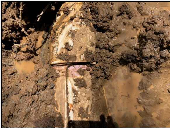
On left you can see the spilt going into the coupling on the right is the completed section with 4" C900 with 45 degree fitting.
