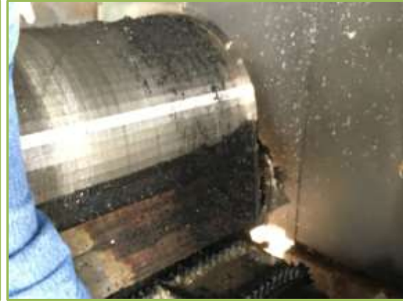
Sand and Debris that plugged the inlet to roto drum #2
