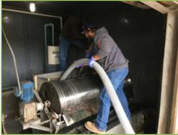
Sand and Debris that plugged the inlet to roto drum #2
