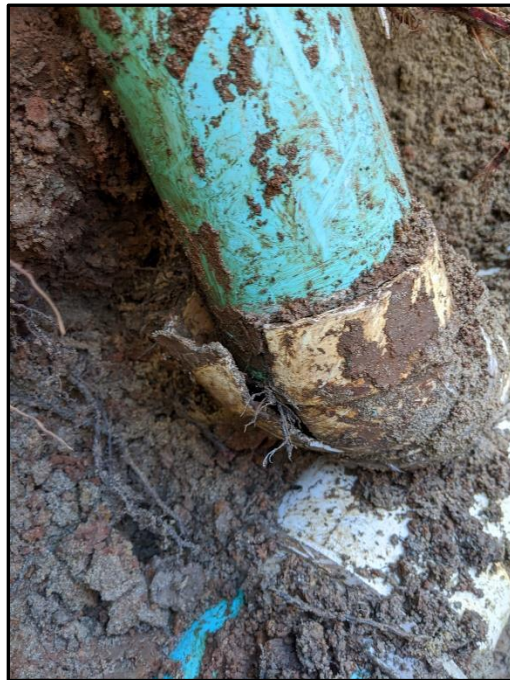
Repair Root intrusion at broken lateral fitting
