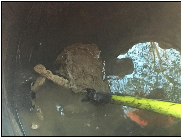
Root ball and grease broken lose from Hydro Flushing left Root ball and grease removed right
