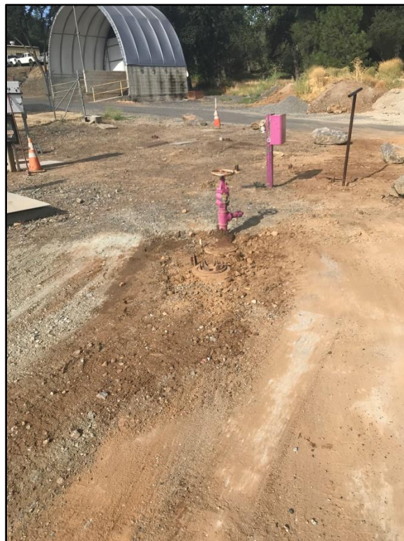
Bonnet was removed and seat was replaced with parts found in Bone yard dated 1979
