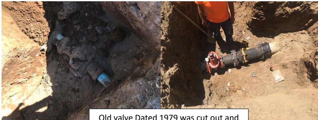
Old valve Dated 1979 was cut out and replaced with new section. Valve was stuck in the open position
