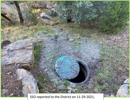
Manhole was located below Lower Skyridge Rd, cause was grease flushable wipes/rags
