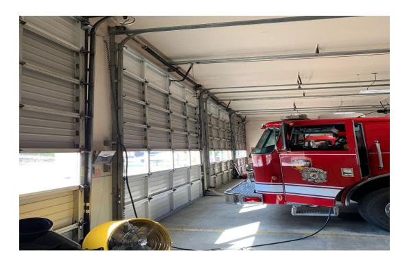
We received great news that our FEMA Assistance to Firefighters Grant Application from 2021 was approved. We applied for funding for a Plymovent exhaust system, which removes all of the vehicle exhaust from all vehicles within the apparatus bay at station 78, and it exhausts it through the roof. We were awarded \$41,336.23, and GCSD is responsible for paying \$2,066.82. This is an amazing station upgrade.
