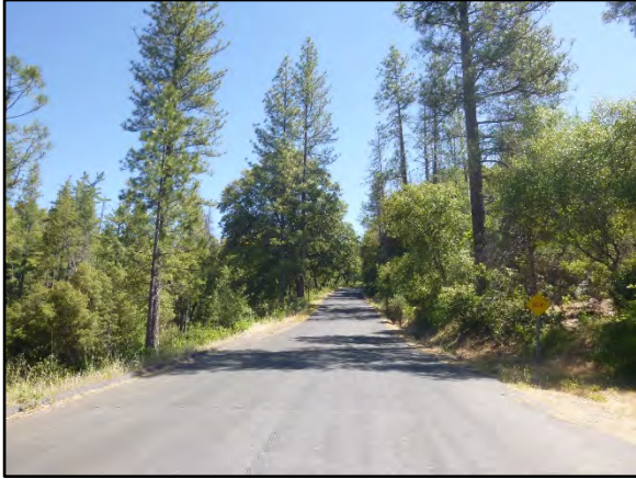
Photo 7. View N, replacement water main route at Hwy 120 & Whites Gulch R.
