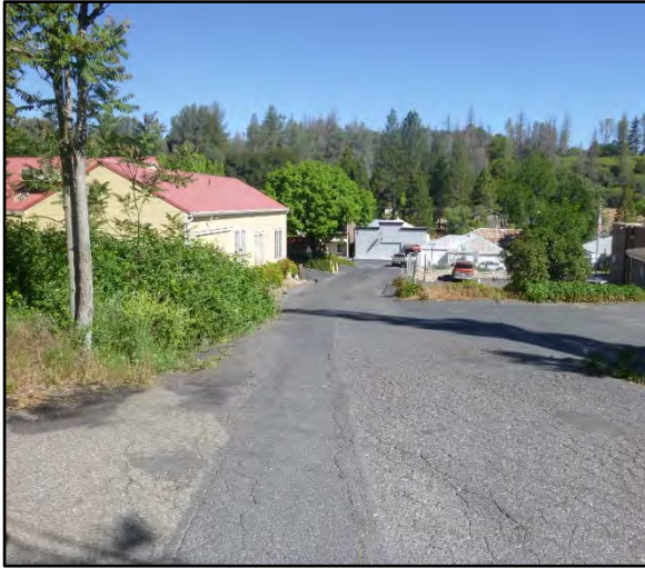
Photo 3. View NW, new water main route at Powder House & Foot Streets.
