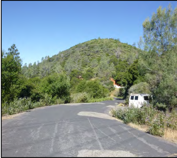
Photo 1. View W, new water main route at Big Oak Rd & Wards Ferry Rd.
