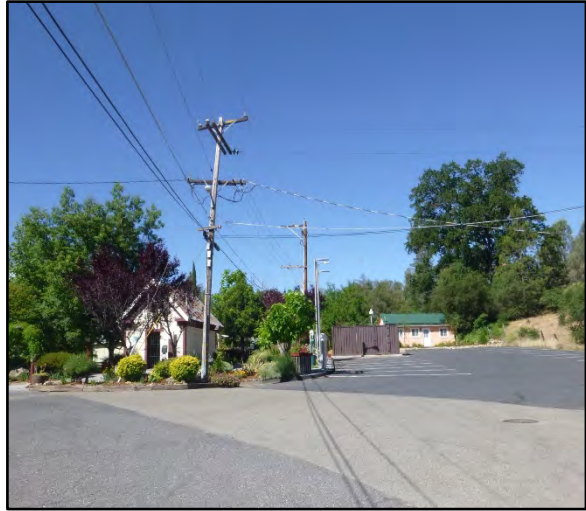
Photo 4. View SE, water main route, Ponderosa Lane (note Old Jail structure at center left).
