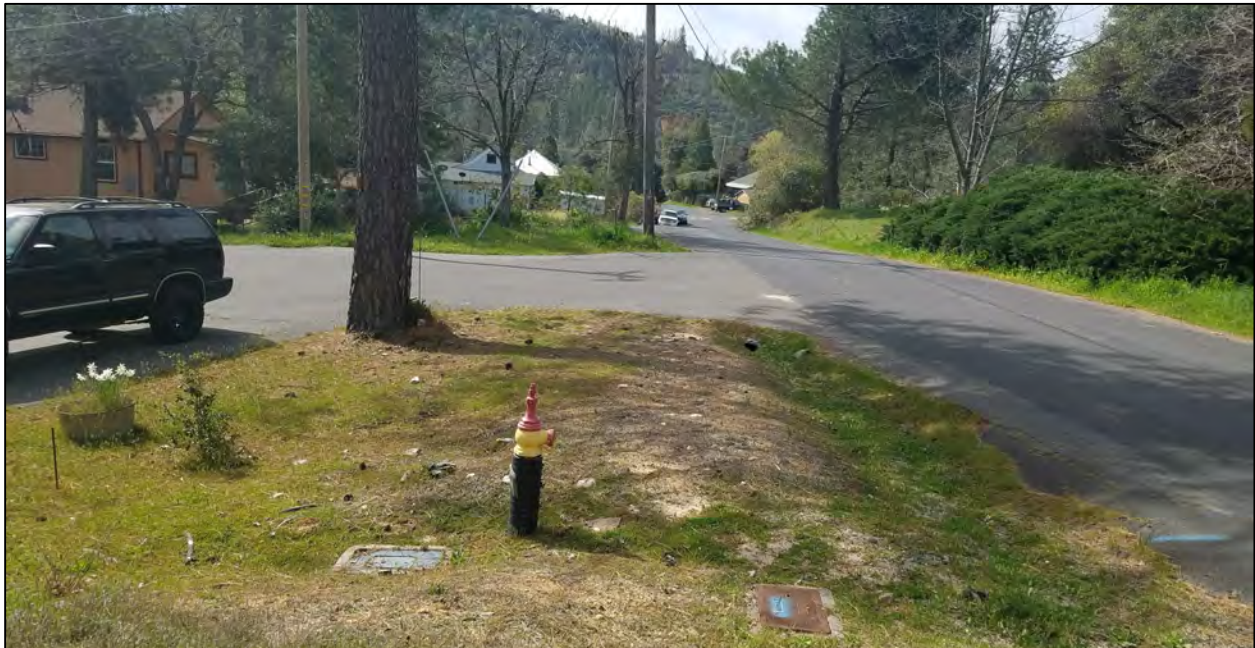
Figure 6. Photograph of the Big Oak Flat Project location showing existing water main infrastructure in developed and disturbed land cover surrounded by cismontane woodland.
