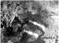
Possible water break unit 1 lot 312 due to suburban propane truck running over meter box. District lines were ok both PO lines were broke.
