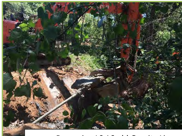
Removing LS 16 old Gravity Line
