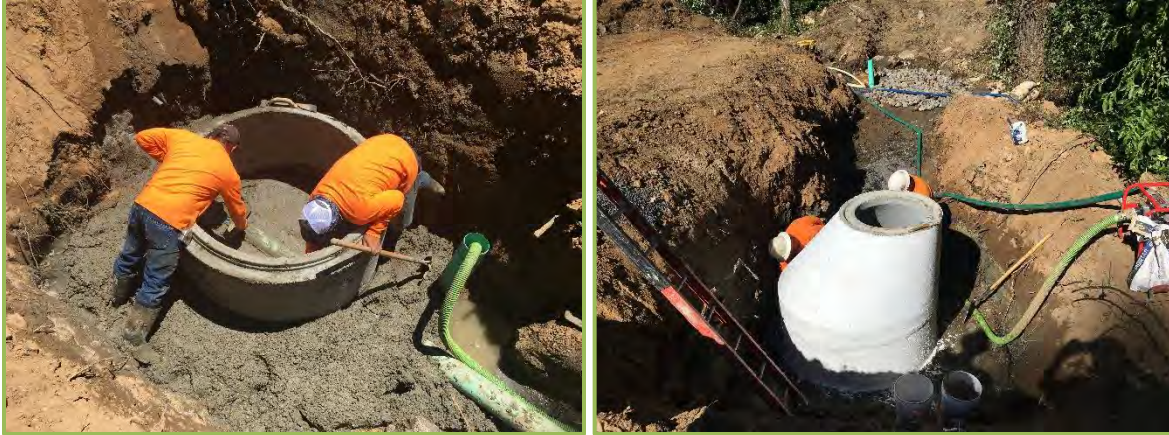
Installing new pour in place Manhole
