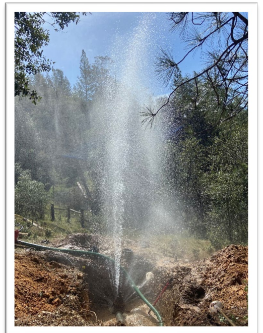
Dewatering the mainline for valve replacement.
