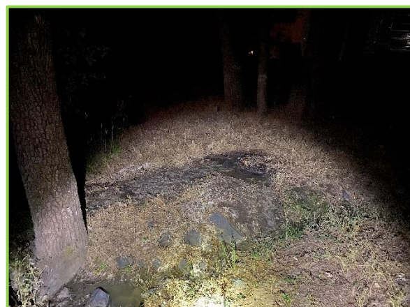
Manhole Spilling due to root blockage
