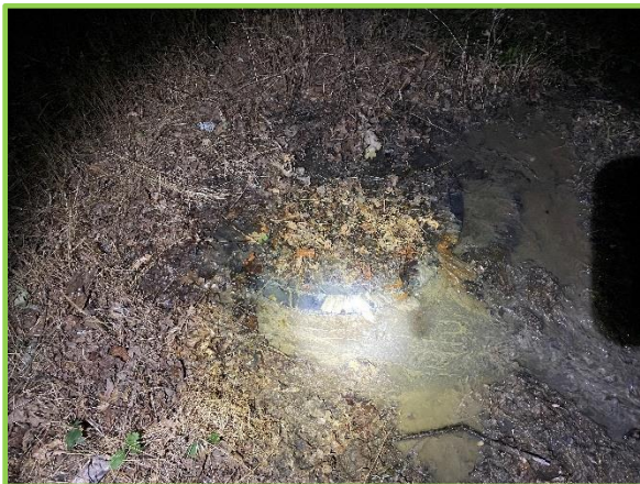
Manhole Spilling due to root blockage
